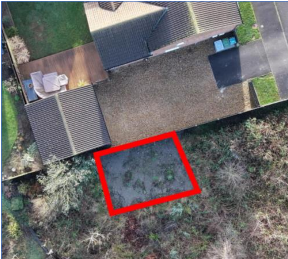
Compliance Drone Photo
